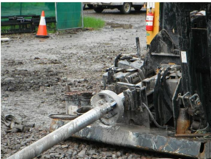
1/2" went successfully with only 1 chipped PDC. General ROP was 13 min/rod on 6.1m rods at 50RPM. The overall consensus was that the reaming was highly successful enabling pipe pull within 2 weeks of starting the process.
